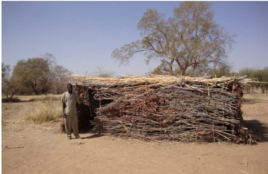
The Headmaster of Koutougou Primary School next to one of two temporary classrooms currently accommodating some 40 students. Middle Island intends to construct two new classrooms as part of its social development initiative at Nassilé for 2011/12.
