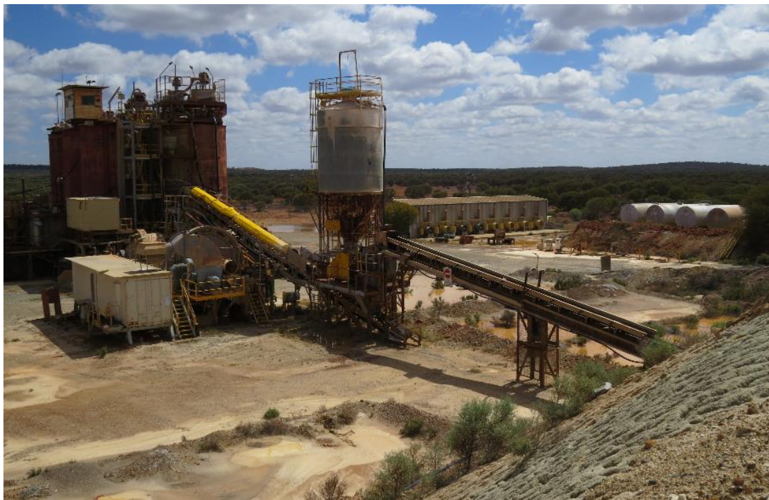
Figure 1 View of the plant from the ROM pad
