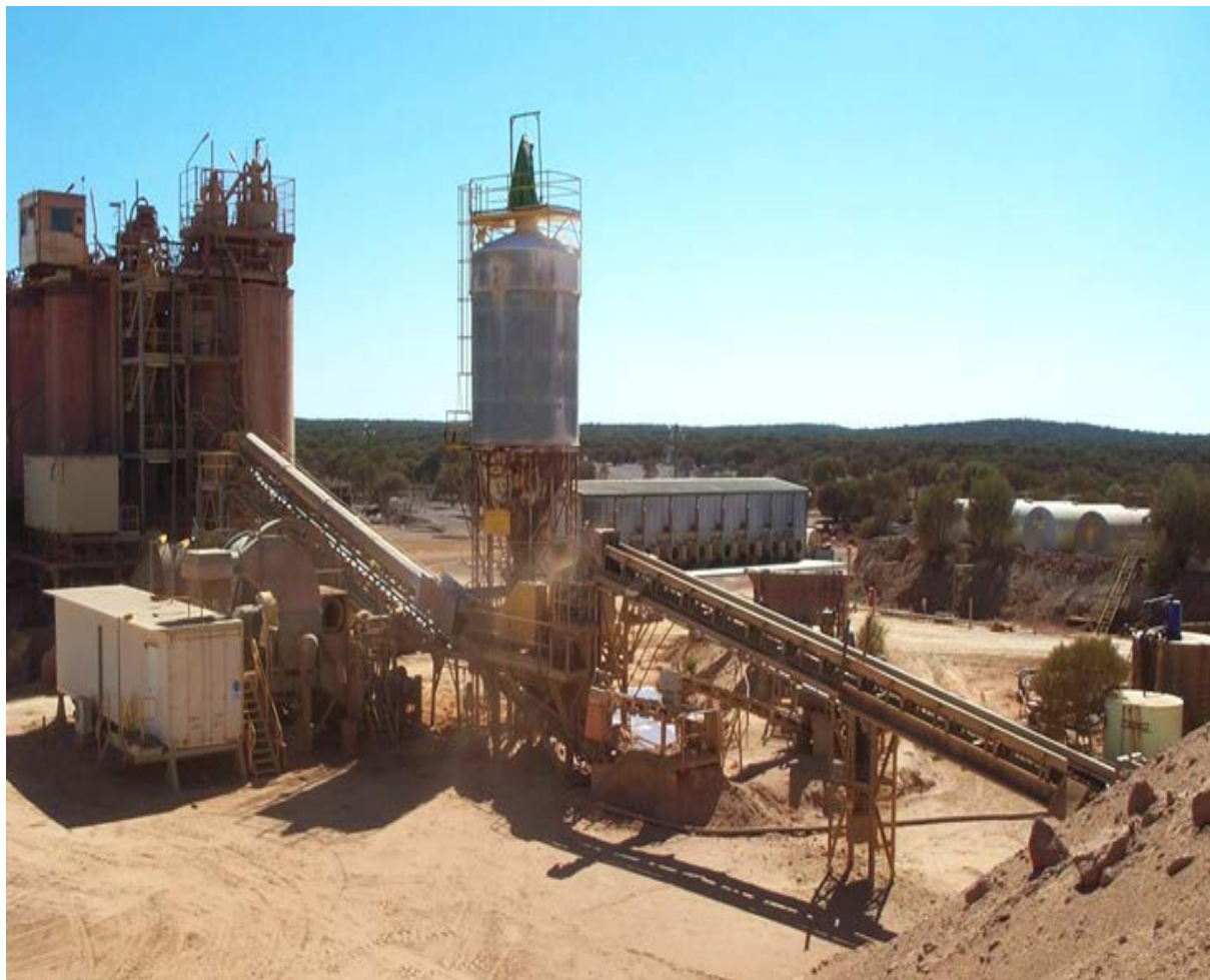
Figure 2 Sandstone processing plant with power plant and fuel tanks in the background
